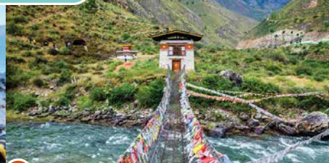
Suspension Bridge 悬索桥
